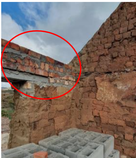
Fig 18 – Raised side walls (supplied by author)
