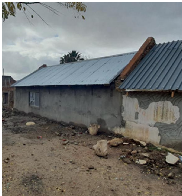
Fig 19 – Consequence of raising side walls (supplied by author)
