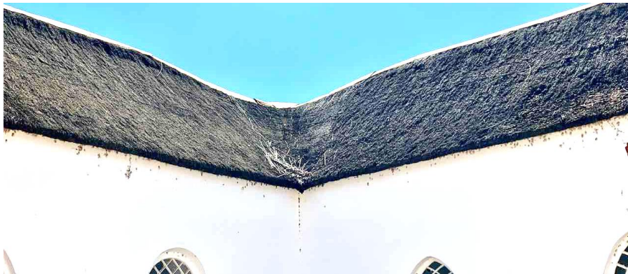
Figure 16A: View of the thatch roof of the church before reconstruction. The roof was in very poor condition and in a state of near collapse between nave and transept. (Image: ARCON, 1 Nov. 2019)
