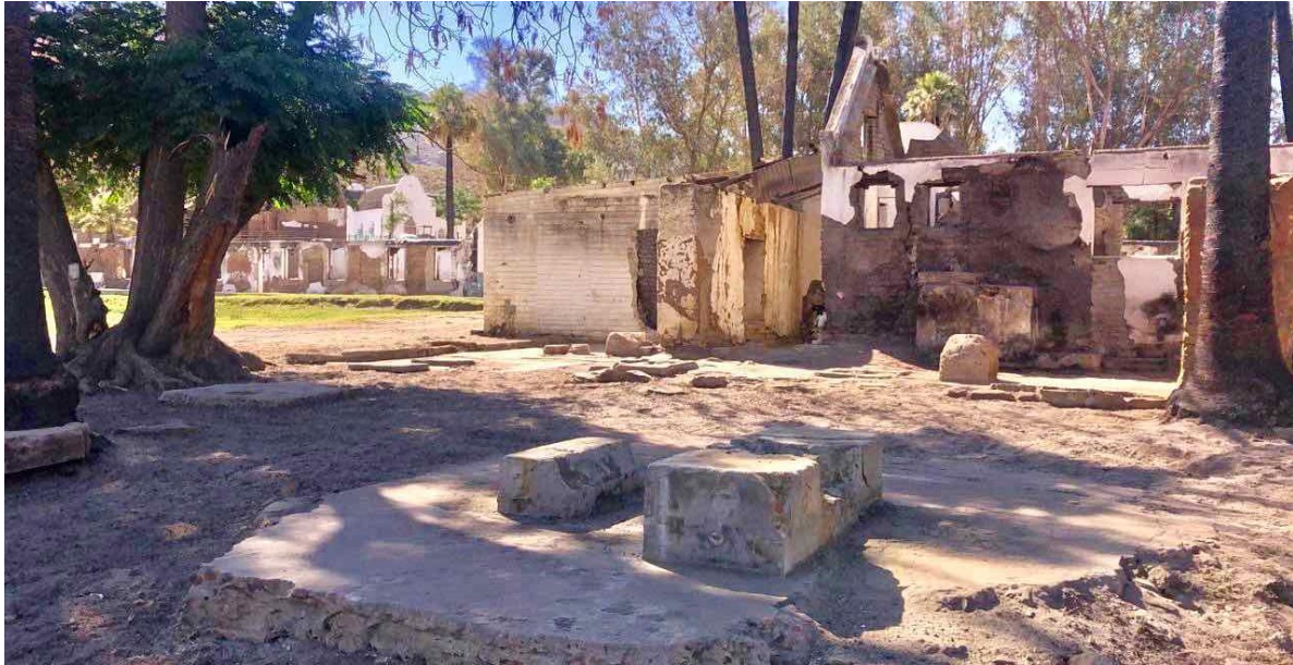
Figure 19D: View of the back of the tannery after the fire (southwest end) showing various remnants of cement and concrete bases which once supported tanning machinery. The 'stoep' in the foreground was once under a lean-to roof, and remains of an old stone wall base are visible running diagonally across the foreground (Image: ARCON, 6 December 2019)
