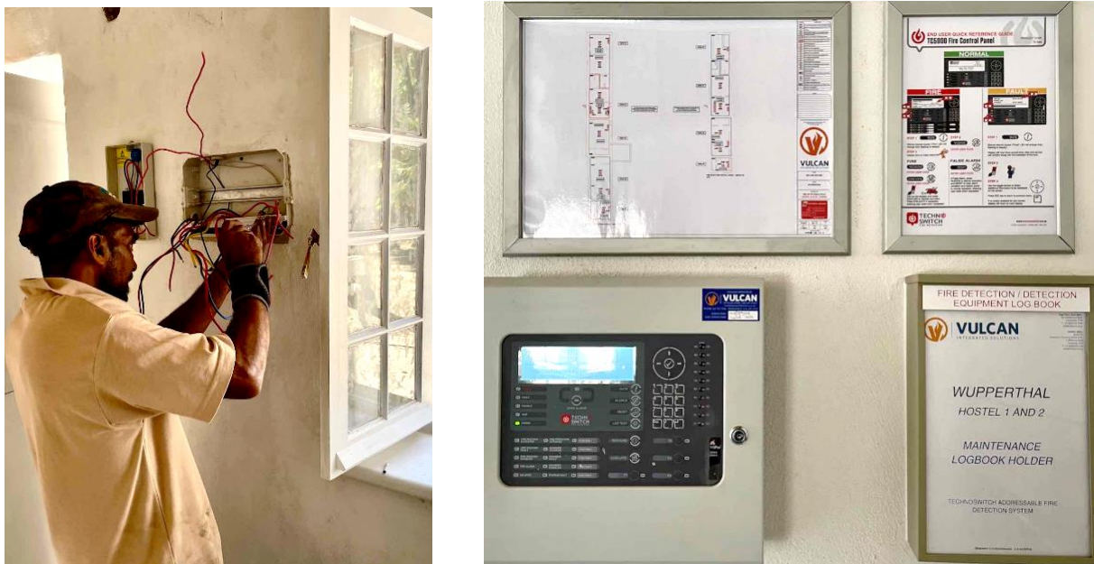
Figure 23E: New fire sensor and alarm systems were installed in all the restored buildings. Prior to the fire, the only alarm system in the settlement had been the church bell. (Images: ARCON, 7 April 2021)
