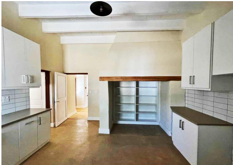
Figure15F: New simple, contemporarily styled kitchen with reconstructed hearth converted to a pantry. (Image: ARCON, 7 April 2021)
