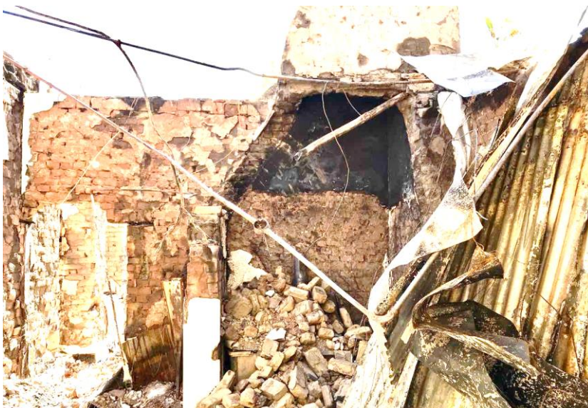
Figure 15E: Collapsed kitchen hearth in the Winkelhuis after the fire. All intact bricks were recovered and re-used in its reconstruction. (Image: ARCON, 24 January 2019)
