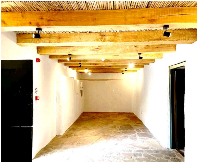
Figure 23F: New fire alarm system in Leipoldt House. The panic button and red alarm light are next to the front door (left) with the control panels at the left far end. Smoke detectors are mounted to the underside of new rafters supporting a new brandsolder and reed ceiling. (Images: ARCON, 8 June 2021)
