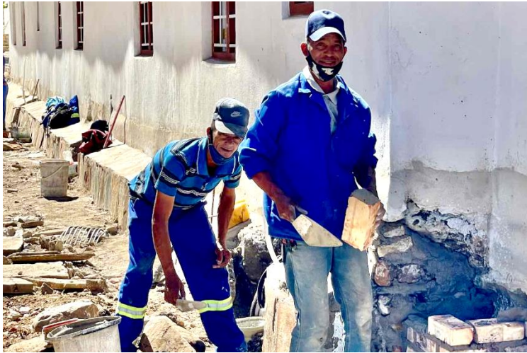
7 April 2021: Wall repairs at the back of one of the School Hostel buildings. The mortar has the appearance of Portland cement but is actually builder's lime mixed with a very dark local river sand.
