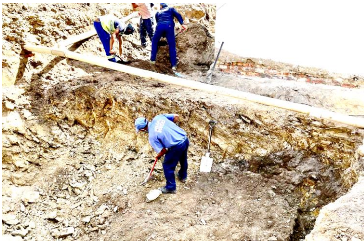
9 March 2021: Digging the massive new underground sump behind the School Hostels as part of a system to alleviate future stormwater flooding.
