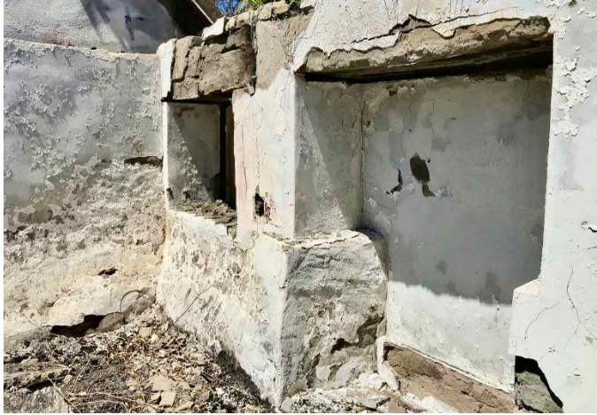
Figure 21C: A portion of the gutted interior of the Palms Guest House after the fire. (Image: ARCON, 24 January 2019)
