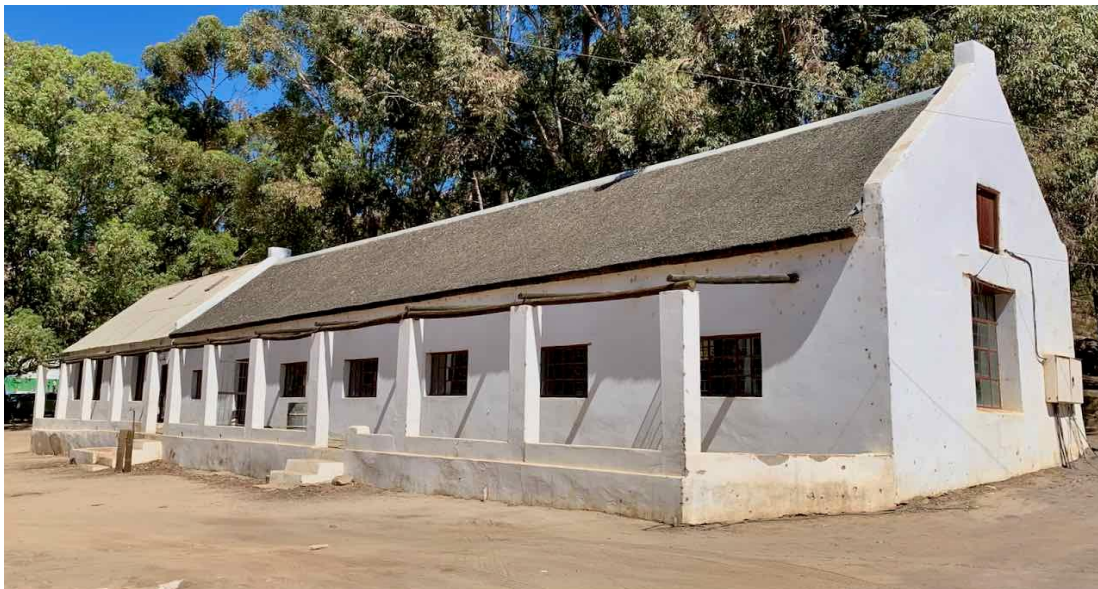
Figure 18D: Exterior of the shoe factory prior to refurbishment. It had been re-thatched by the Moravian Church a few years previously. The extension on the far left was then used as the town library and had a corrugated iron roof. (Image: ARCON, 17 March 2020)
