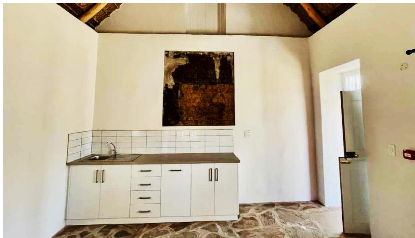
Figure 28B: Masonry panel left unplastered and treated with a special breathable fixative to prevent it from dusting. This panel shows three periods of construction with a partly charred lintel from the fire still in place. This image was taken before the interpretative plaque was fixed to the wall. (Image ARCON, 14 January 2021)
