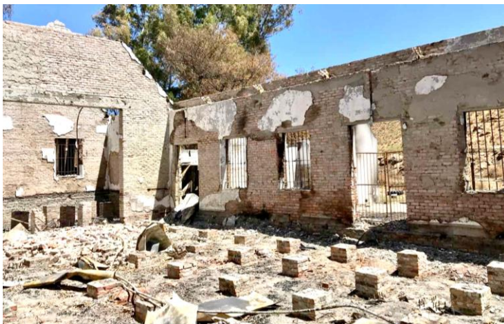
Figure 11C: Gutted interior of the Community Hall after the fire. (Image: ARCON, 24 January 2019)
