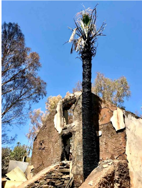
Figure 23B: Palms were likely the most instrumental in spreading the fire in the Church Precinct due to the aeration imparted by the shape of their fronds. Although palms strongly characterize the precinct, these and other trees close to the thatch buildings had to be removed as a precaution against the spreading of future fires. This example would have been at least partly responsible for the gutting of Leipoldt House. Its removal was debated at the time because of the risk its removal posed to the foundations of this historic building. Ultimately, it was removed, and a small buttress constructed to reinforce the base of the wall in its place. (Images: ARCON, 24 February 2019 & 23 March 2021)
