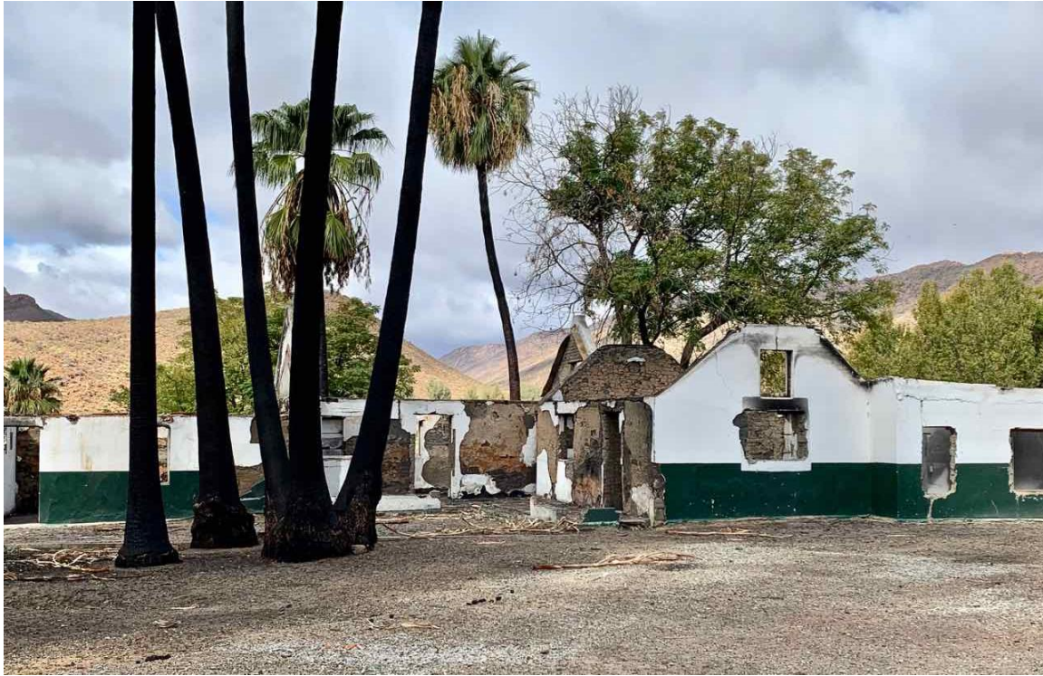
Figure 19A: The Old Tannery after the fire. Burning palm fronds played a large role in spreading the fire in the strong wind that had prevailed. (Image: ARCON, 26 May 2020)
