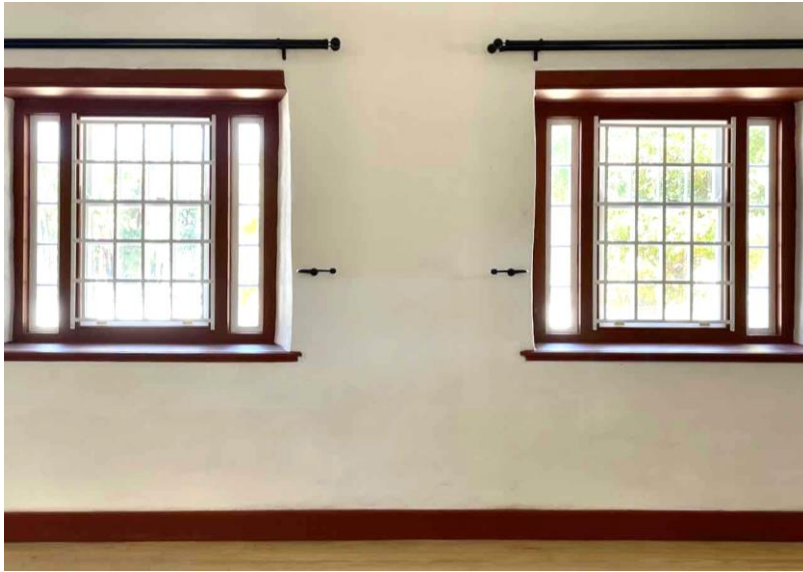
Figure 13F: Replacement windows in the Mission Stores after restoration. It is suspected that the additional glazing on the sides was to provide extra light for pupils when the building was still a school in the 1830's. (Image: ARCON, 7 April 2021)
