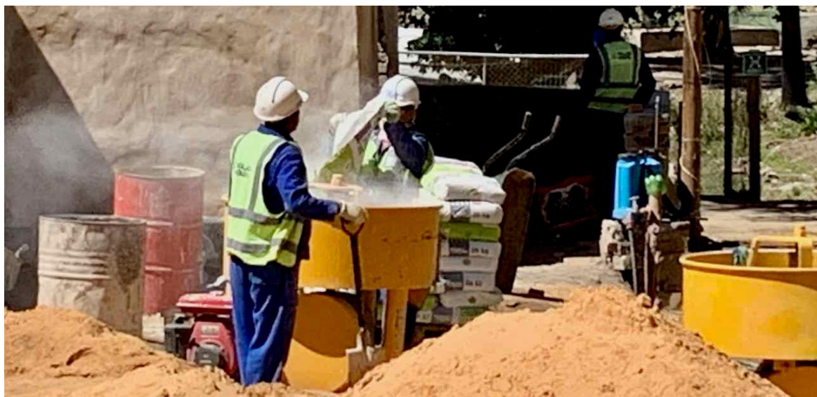
Figure 9: Pan mixers in action preparing lime/sand mortars and renders. The sand used was Malmesbury sand which is coarser and therefore preferred over finer Cape Flats silica sands for work on historic buildings. (Image: ARCON, 25 October 2019)
