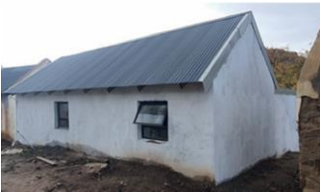
Figure 20: Side walls raised and gables covered over. (Author)
