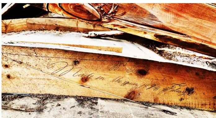
Figure 16C: Carpenter's signature on one of the saucer vault ribs record that the ceiling was added in 1894. This practice has been revived at Leipoldt House and other new joinery forming part of the restoration process (Figure 10F). (Image: ARCON, 1 Nov. 2019)
