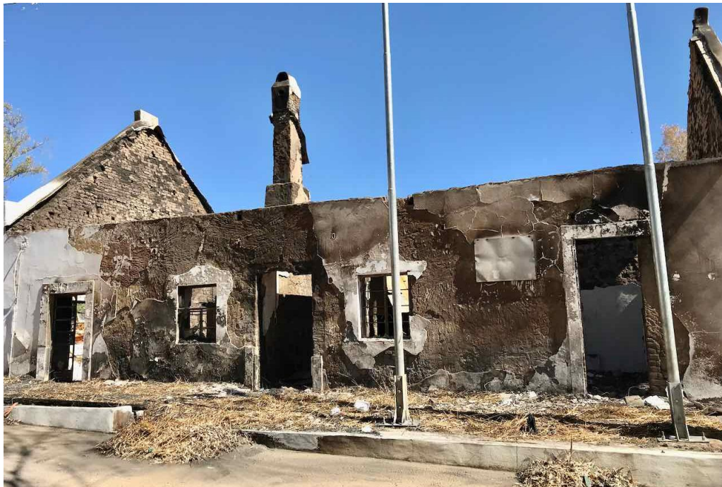
Figure 3: The fire-gutted 'Winkelhuis' (Shopkeeper's House) after the fire. The building had been the administration headquarters for the town before the fire. This image is typical of the degree of damage sustained. (Image: ARCON, 24 January 2019)
