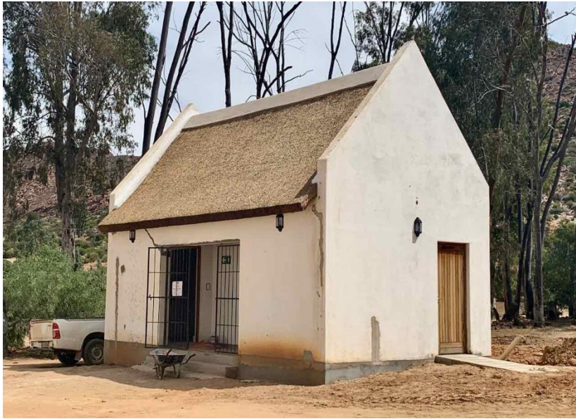
Figure 24B: The church ablution after re-thatching and undergoing crack repairs prior to repainting. (Image ARCON, 27 October 2020)
