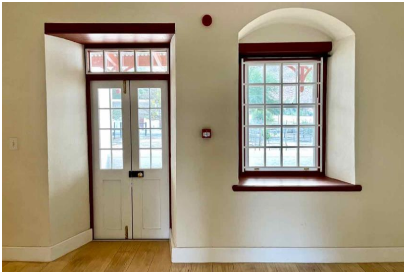
Figure 15D: The same view as Figure 15C after restoration. The door opening on the left had to receive a horizontal lintel after the previous segmental arch suffered a collapse. (Image: ARCON, 16 October 2020).
