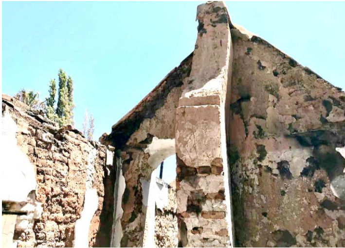
Figure 22C: The remains of the forge flue after the fire. (Image: ARCON, 24 January 2019)
