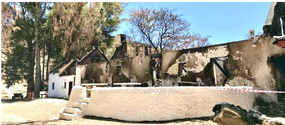
Figure 10A: : Exterior of Leipoldt House after the fire. This building is most probably the original Rietmond farmhouse, pre-dating the arrival of the Rhenish missionaries by about 30 years. The uncharacteristic semicircular stoep appears to have been used as a podium from which open-air services were conducted before the church was completed, explaining its non-traditional shape. (Image: ARCON, 25 October 2019)
