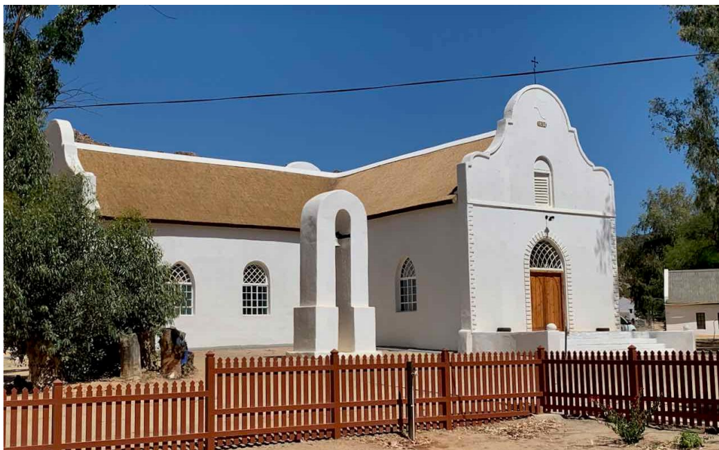
Figure 16F: The church building after completion of the new roof and repainting with a propriety breathable wall coating. (Image: ARCON, 14 January 2021)
