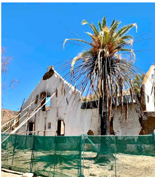
Figure 23C: Left: A palm next to the Winkelhuis was another example of a tree removed for fire security reasons. This image also indicates the emergency propping installed shortly after the fire using locally available timber to prevent a gable collapse. Right: the size of the root bowl of the palm after its removal. (Images: ARCON, 24 February 2019 and 11 October 2019)
