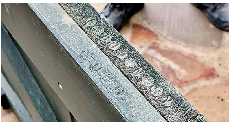
Figure 10F: Carpenter's marks: All new joinery in Leipoldt House and other buildings was stamped with the name of the joiner and date of fabrication in inconspicuous places as a record for future researchers: all in the tradition of historic carpenter's marks incised into their work through the ages, and consistent with similar early practices in the town (see Figure 16C) (Image: ARCON, 8 June 2021)
