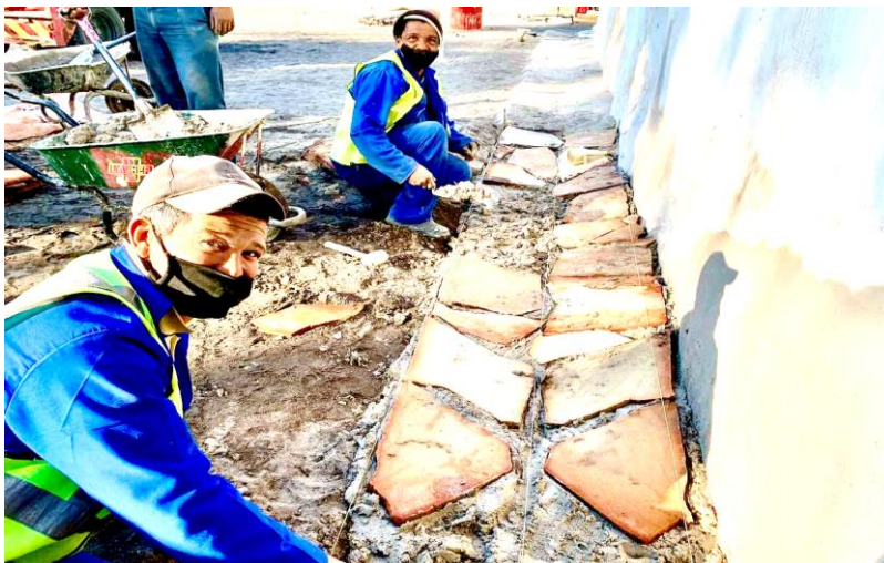
6 August 2020: Laying new rainwater channels for Leipoldt House.
