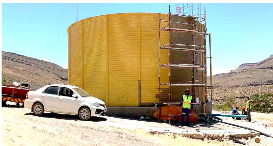
Figure 27A: The new reservoir funded by the Foundation nearing completion. (Image ARCON, 14 January 2021)
