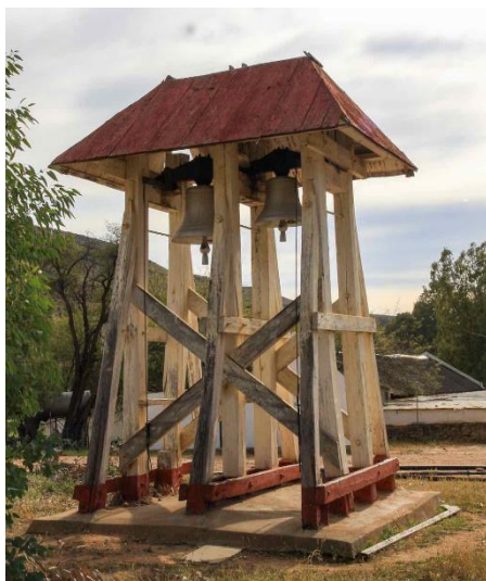
Figure 24A: The campanile behind the church. Left: before refurbishment. Right: the campanile after refurbishment. The stays had been added by the locals at some stage after the 2009 photograph on the left and did not form part of the restoration project. (Image left: Gabriel Fagan Architects, 22 September 2009; right: ARCON, 27 October 2020)
