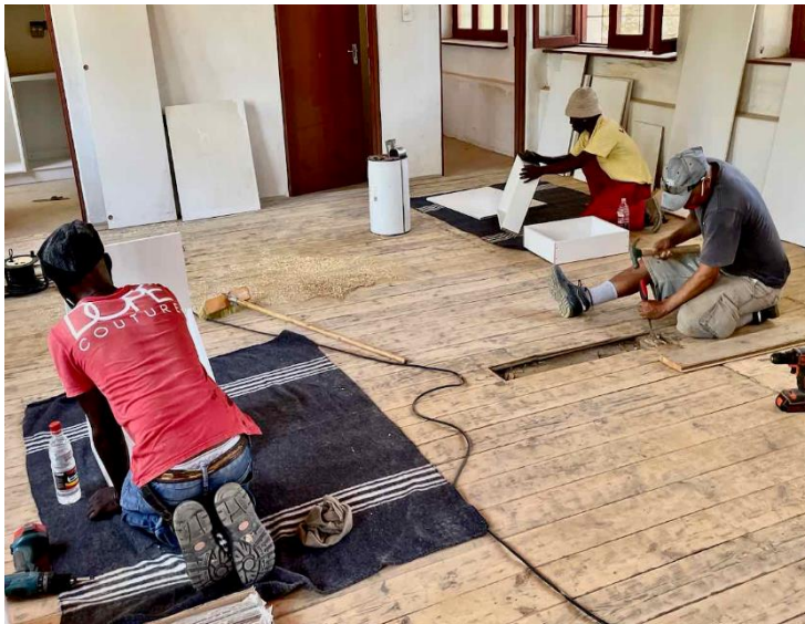
23 March 2021: Repairing the floor in the new Shoe Factory shop space.
