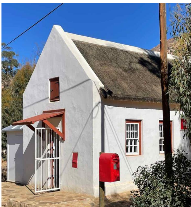
Figure 17B: The Post Office Building after refurbishment including new paving on the front stoep using locally sourced sandstone laid by local labour. A smaller corrugated iron front entrance canopy replaced the previous burned-out thatch canopy which had too shallow a pitch to withstand protracted weathering. (Image: ARCON, 18 May 2021)
