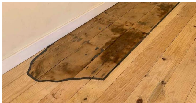
Figure 15G: Remnant of cedarwood flooring recovered after the fire and set into the new floor in the same position where it had been recovered. An interpretative plaque explaining the significance of these floorboards has been placed on the wall above. Out of all the buildings damaged in the fire, this is the only area where a small portion of cedarwood flooring survived. (Image: ARCON, 27 November 2020)
