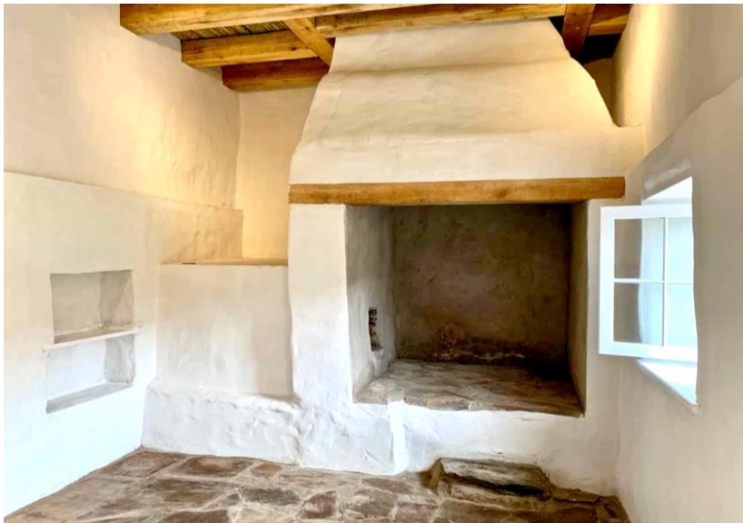
Figure 10D: The kitchen of Leipoldt House after restoration and reconstruction of the hearth flue. (Image: ARCON, 1 September 2020)
