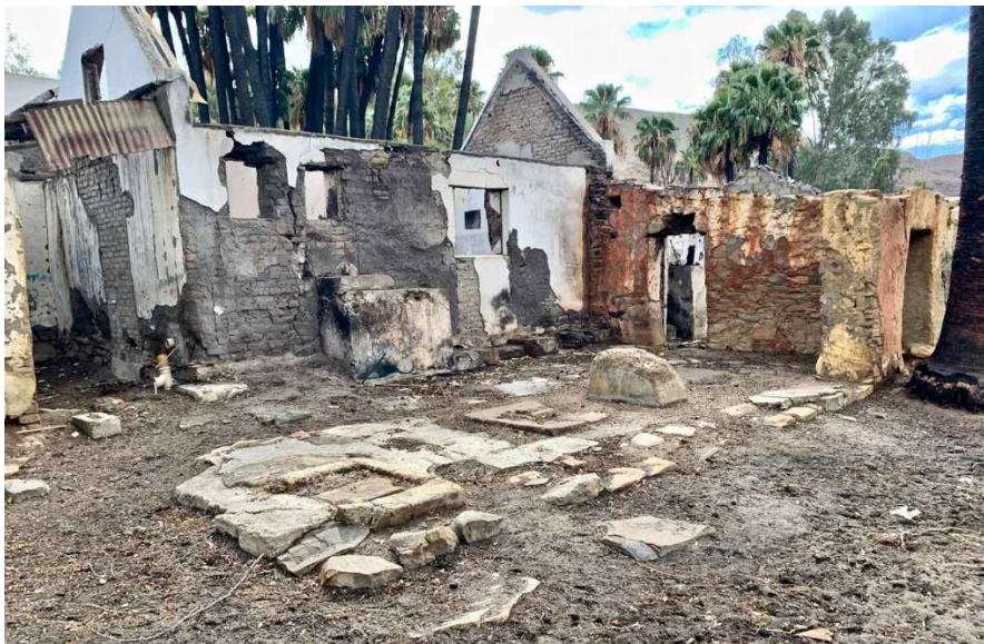
Figure 19D: View of the back of the tannery after the fire (southwest end) showing various remnants of cement and concrete bases which once supported tanning machinery. The 'stoep' in the foreground was once under a lean-to roof, and remains of an old stone wall base are visible running diagonally across the foreground (Image: ARCON, 6 December 2019)
