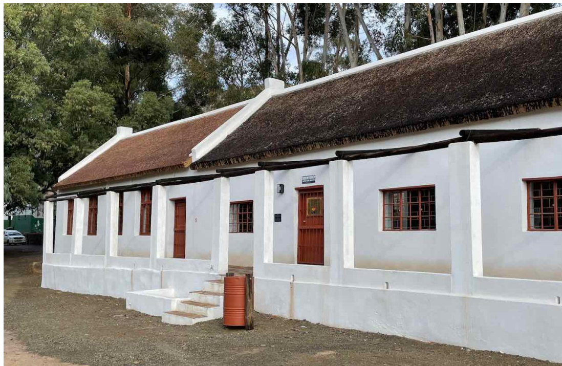
Figure 18E: Exterior of the Shoe Factory after refurbishment. The extension on the far left was provided with a thatched roof to match the roofscape of the rest of the town centre. The interior was refurbished to provide a shop for the factory. The steel windows were retained. (Image: ARCON, 8 June 2021).
