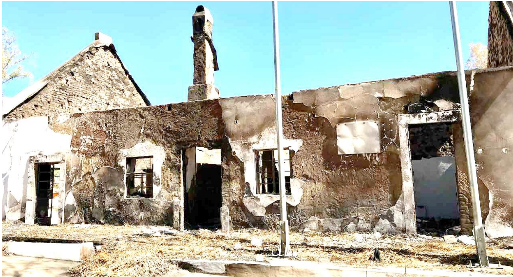
Figure 15A: The front façade of the Winkelhuis after the fire. This was one of the buildings initially considered particularly dangerous with various large wall cracks. However, on closer examination, it was found that the cracks pre-dated the fire. (Image: ARCON, 23 March 2021)
