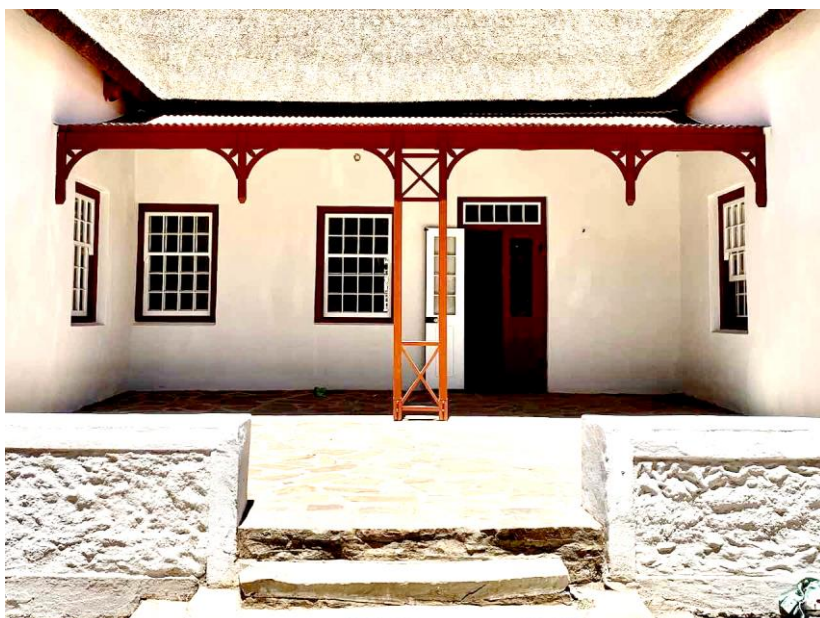
Figure 15H: Rear veranda of the Winkelhuis with reconstructed canopy based on a photograph that the author, by pure coincidence, took on a casual visit to Wupperthal about 4 months before the fire. That photograph proved to be the only known record of the rear façade of the house with its canopy. (Image: ARCON, 27 November 2020).
