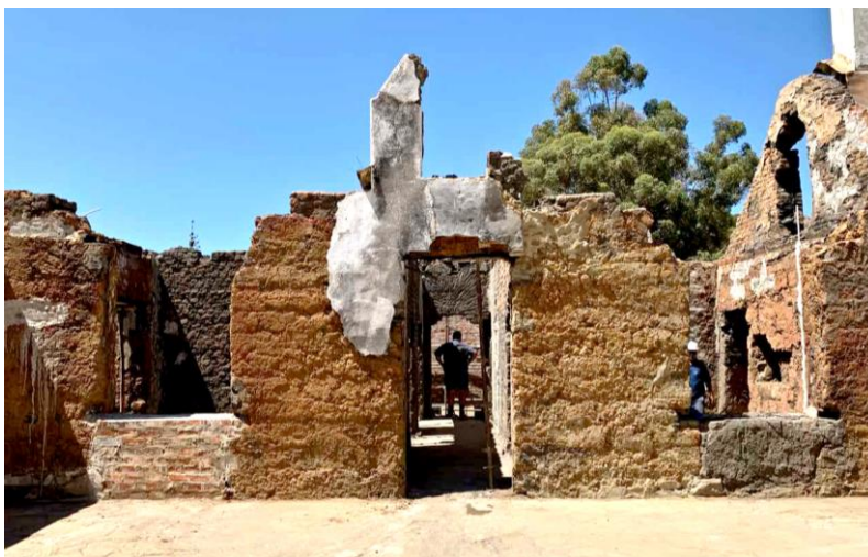
Figure 14C: The front façade of the Parsonage after the fire debris had been cleared. The rammed earth construction of the central portion of the facade is clearly evident in the horizontal wall striations. (Image: ARCON, 30 January 2020)
