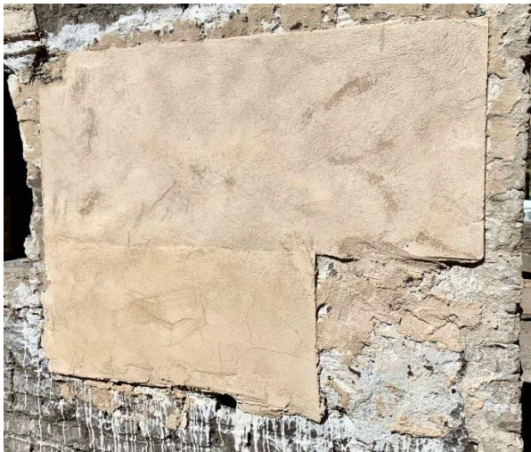
Figure 8: Trial panels using lime/sand mixes for plastering and laying brickwork. Left: Two separate lime plaster panels experimenting with water proportions. The shrinkage cracks in the lower panel show that too much water was added. Right: Trial samples of brick walls constructed using exclusively lime/sand mortars to convince an initially sceptical contractor that such lime mortars without Portland cement would be structurally sound. The wall in the foreground is constructed using modern fired bricks. The darker wall in the background experiments with bricks recovered from the fire damaged ruins. (Image ARCON, 30 August 2019)
