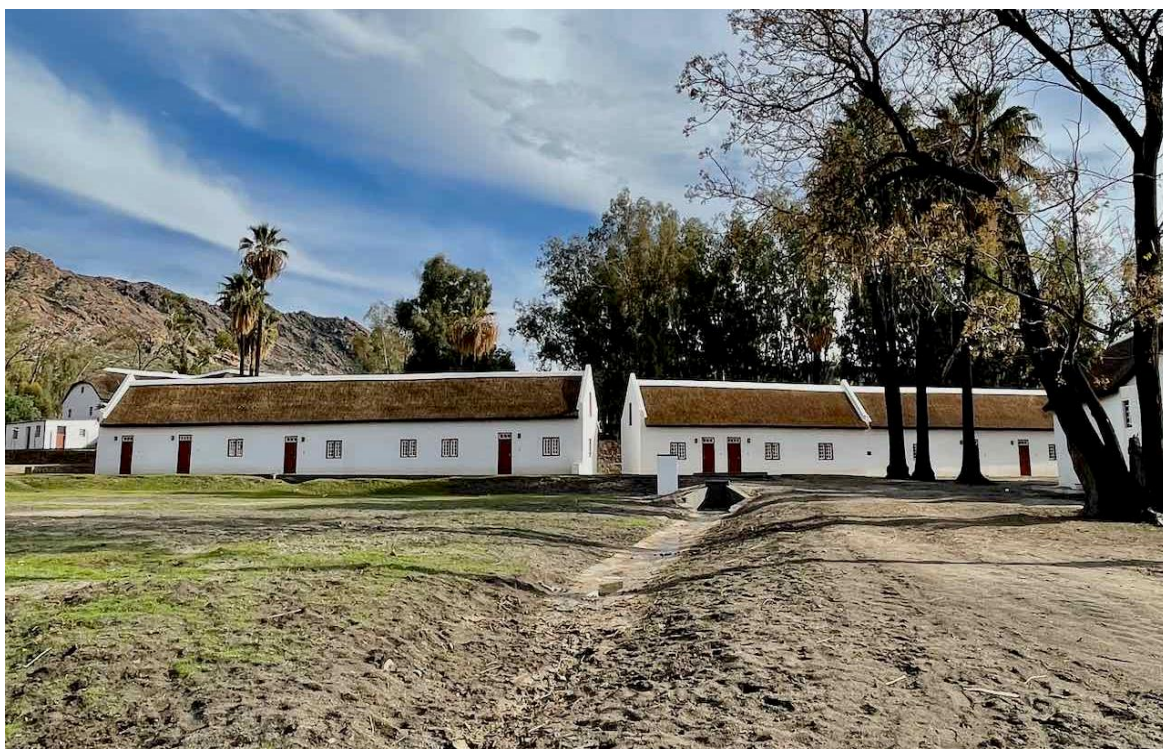
Figure 20F: View of both restored hostel buildings now repurposed as guest accommodation for the village. The channel and outfall in the centre of this image is part of a new stormwater system installed by the Foundation to control flood waters which had previously been a problem, after heavy rains. (Image: ARCON, 4 May 2021)
