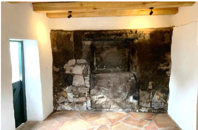
Figure 10E: : Leipoldt House memorial wall: It was decided that one of the end walls in Leipoldt House should be retained in the condition in which it was found after the fire to commemorate the disaster. This was considered especially relevant as this part of the building is scheduled to become the town's museum. (Image: ARCON, 8 June 2021)
